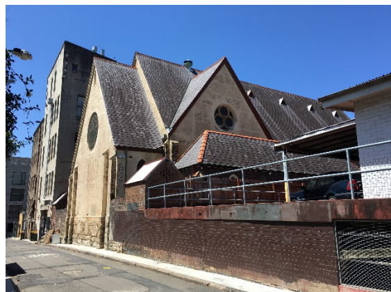
Picture 4 – View of Elizabeth Lane street interface
