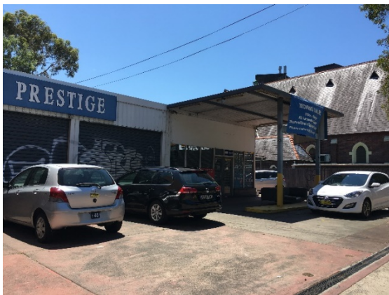
Picture 1 – Existing structures on site
